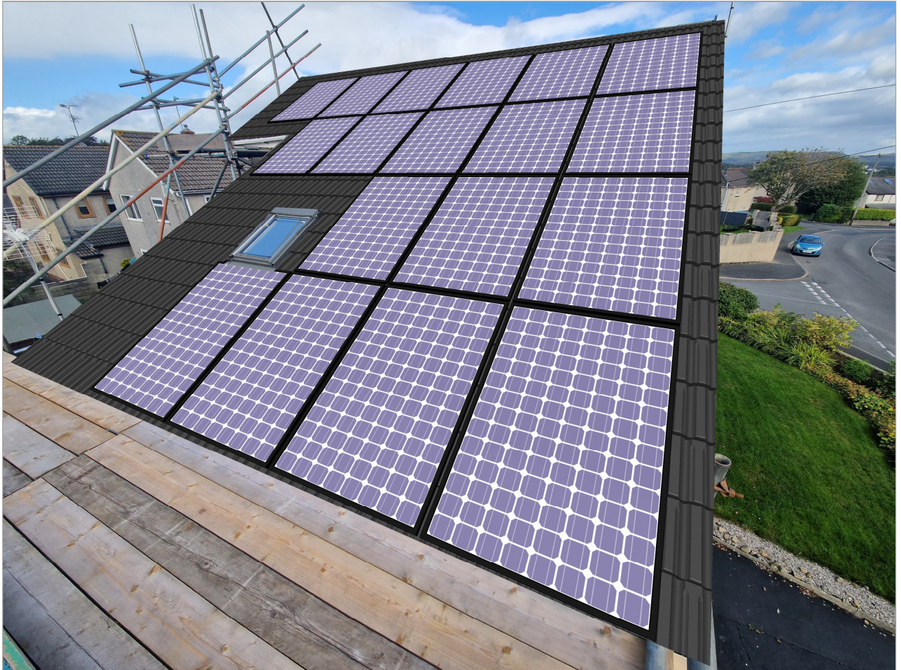
Figure: Photo Preview, 1. Module Area - Module Area 1
