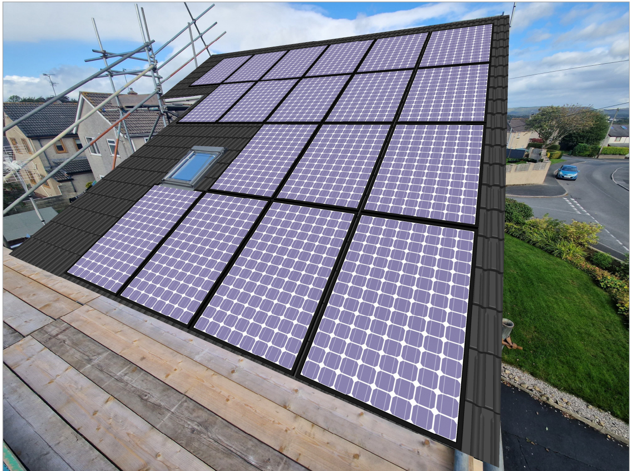
Figure: Photo Preview, 1. Module Area - Module Area 1
